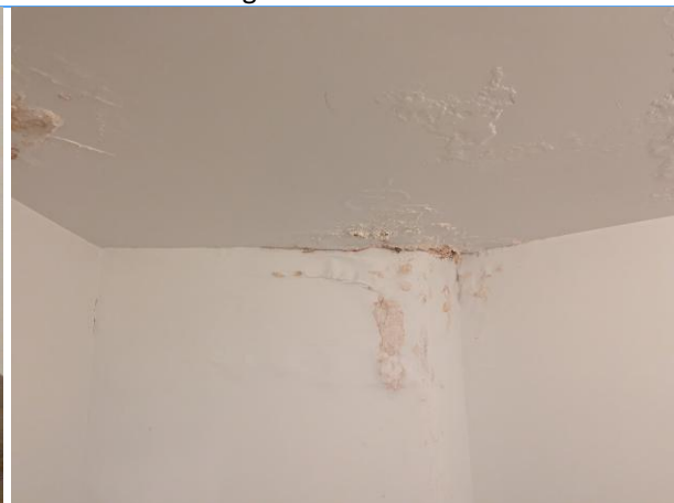
View of the typical water and mold impacted interior finishes in the basement level of Unit 1.
