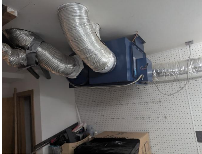
General view of the electrically powered "Environment Air" HRV serving the building.
