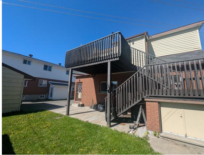
General view of the wooden framed deck located adjacent to the east elevation of the building.
