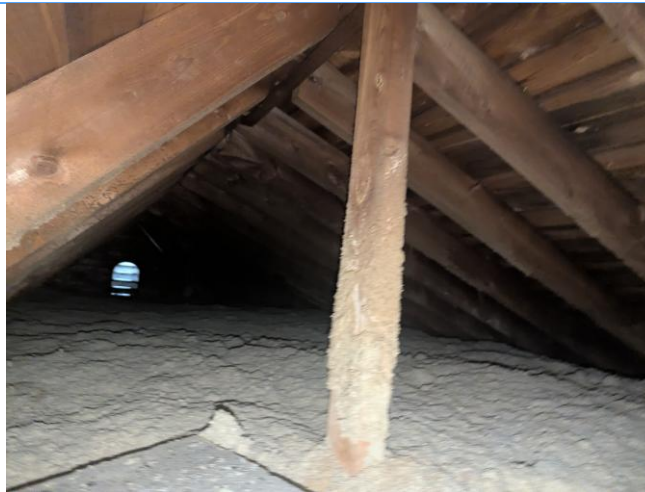
General view of the attic space serving the building.
