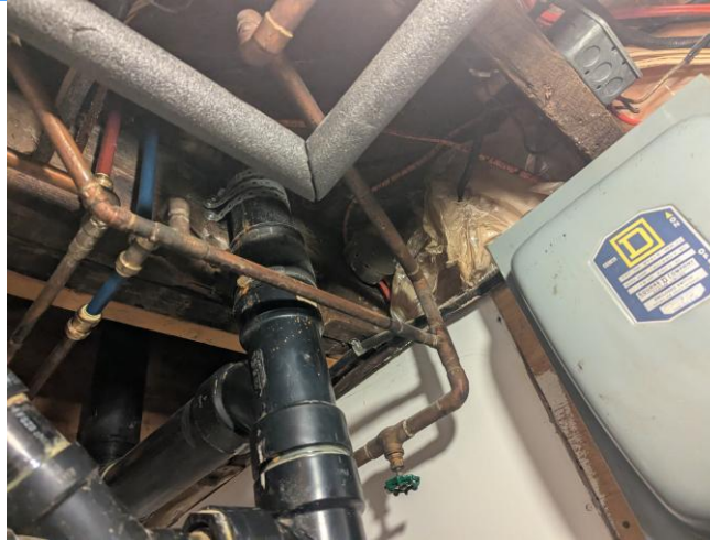
General view of the wooden framed intermediate flooring system serving the building.
