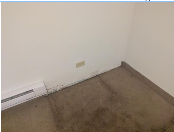
View of the typical water and mold impacted interior finishes in the basement level of Unit 1.
