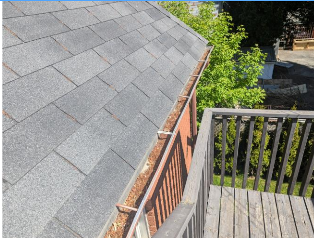
View of the metal eave troughs serving the roof drainage system.
