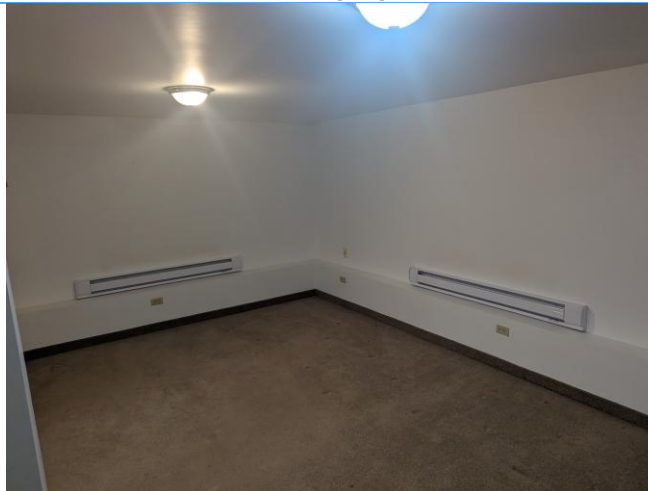
General view of the electrically powered baseboard mounted units serving the building.
