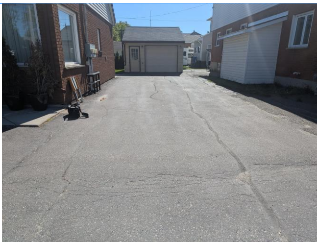
View of the asphalt pavement covered driveway noted on the south portion of the property.
