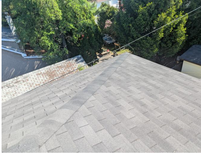
General view of the asphalt shingles serving the roof covering system.
