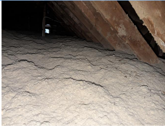
View of the loose fill cellulose insulation serving the attic space.
