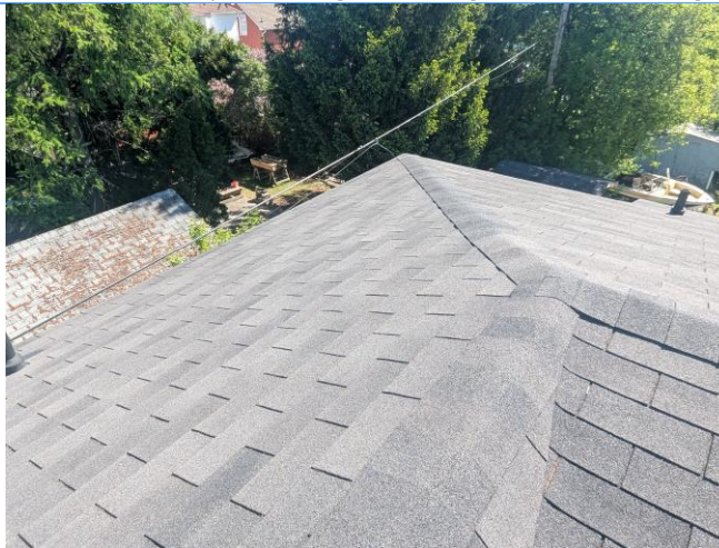
View of the asphalt shingles serving the roof covering system.
