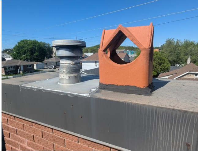
View of the chimney cap serving the roof system.
