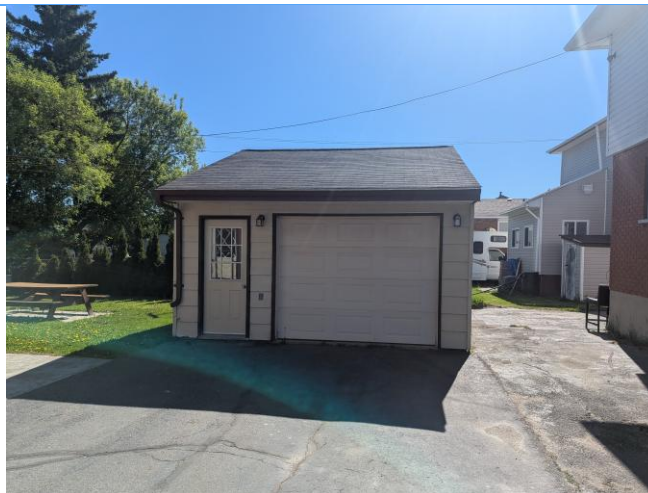
General view of the garage located on east portion of the building.
