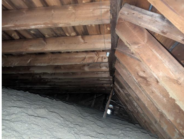
General view of the wooden roof rafter system serving the roof system.
