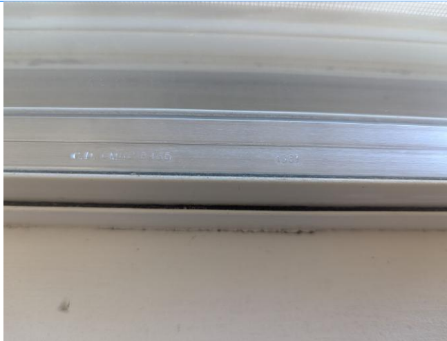
View of the date stamp of ~ 1981 serving the aluminum windows of the building.
