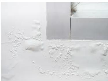
(Bubbled paint over unrepaired water damage)
